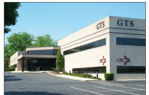
441 Friendship Road, Harrisburg, PA - 57,000 SF high tech office building available for sale and/or lease. 15,000 SF available on the lower level with 19,464 SF available on the first floor. Climate controlled server/computer room. Ample parking. Located in Tecport Business Park. (1879)
