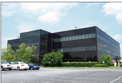
3605 Vartan Way, Harrisburg, PA - 3-story, Class "A" office building for lease. Up to 18,512 SF of contiguous office space available on the first floor with three other smaller office suites available on the 2nd & 3rd floors. High-end finishes throughout. Easy access to I-81, I-83, PA Turnpike, Rt. 322/422 & HIA. (2539)
