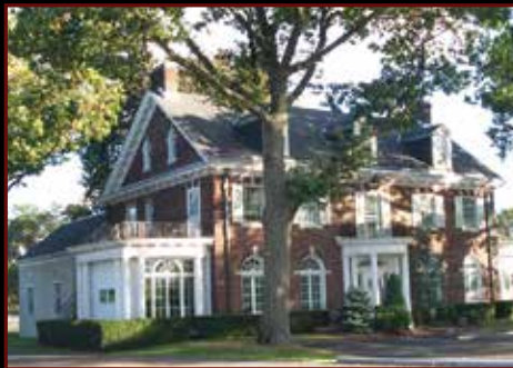
3901 North Front St, Harrisburg 1,397 SF for immediate occupancy. First class finishes. Ideal for any professional
