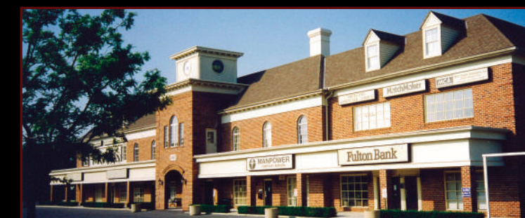
4807-4813 Jonestown Road, Harrisburg, PA 550 to 2,000 SF available for lease. Great signage and visibility. Great suites terrific layouts. Easy access to all areas.
