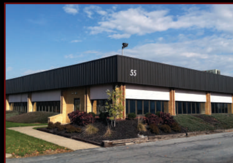
55 Utley Drive, Camp Hill, PA 1,000 to 26,000 SF for lease. New finishes. Ample windows. Convenient Camp Hill address.
