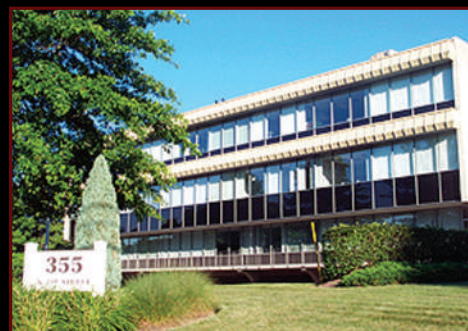
355 North 21st Street, Camp Hill, PA 600 to 3,100 SF available. New suites. Large windows. Covered parking. Great rates.
