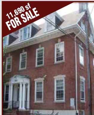
123 Forster Street, Harrisburg, PA
