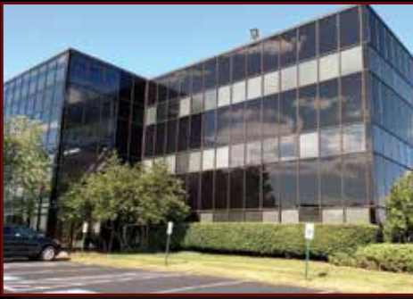
3605 Vartan Way, Harrisburg, PA Suites from 900 to 4,500 SF and up. Terrific windows. Great location. 6 per 1,000 SF parking.
