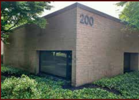
4755 Linglestown Road, Harrisburg PA One suite consisting of 1,359 SF available. Priced to lease. Ready for occupancy.
