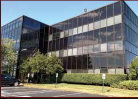
3605 Vartan Way, Harrisburg, PA Suites from 900 to 4,500 SF and up. Terrific windows. Great location. 6 per 1,000 SF parking.
