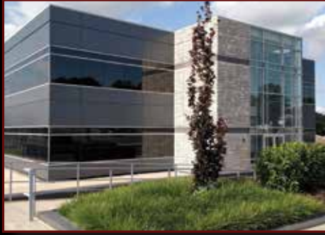
75 South Houcks Road, Harrisburg, PA This gorgeous 29,000 SF first class building offers up to 2,500 SF for immediate occupancy.
