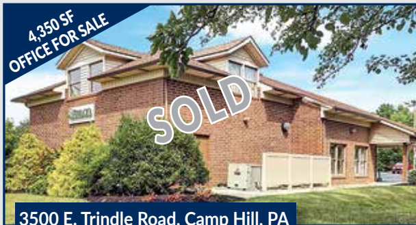
3500 E. Trindle Road, Camp Hill, PA
