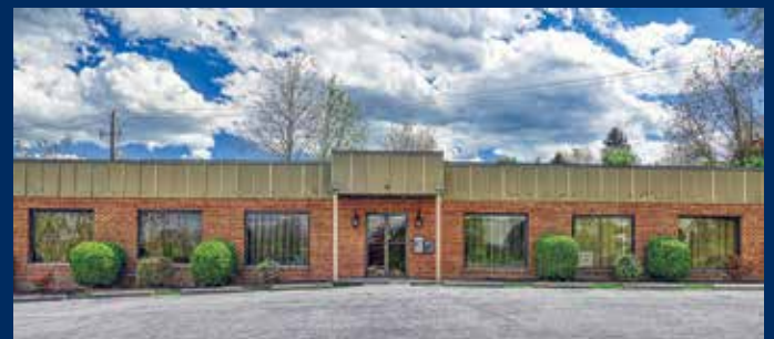
4051 Executive Park Drive, Harrisburg, PA 2000 SF available immediately, just renovated, convenient access.
