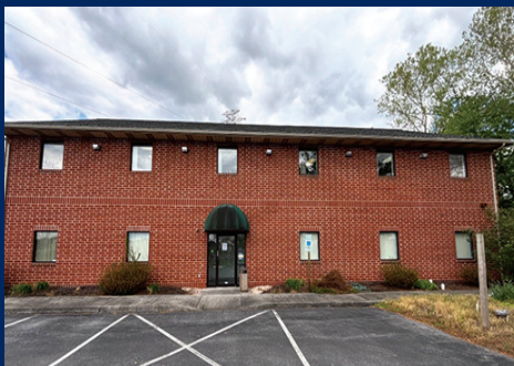
1305 Middletown Road, Middletown, PA Opportunity to lease 4500 SF turnkey dental office just minutes to Hershey.
