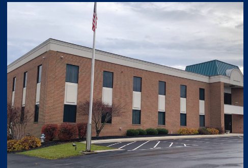
1201 Fulling Mill Road, Middletown, PA New lobby. New finishes. Up to 12,000 SF available.
